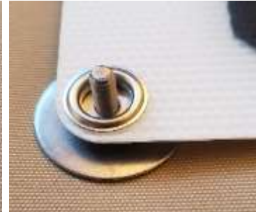
Place washer and panel grommet on bolt
