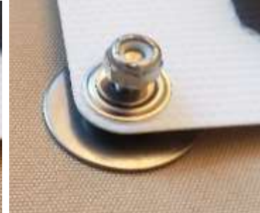
Place washer and tighten lock nut
