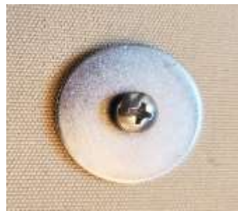
Insert bolt with washer
