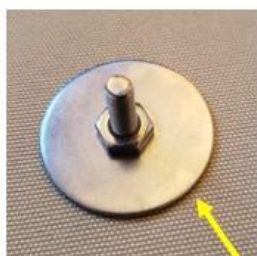
Apply optional adhesive Secure washer with nut
