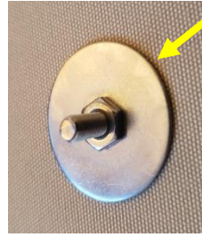
Apply optional adhesive Secure washer with nut
